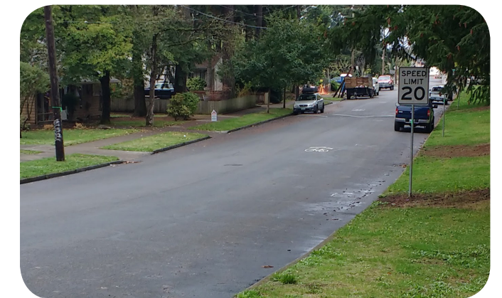
Typical 20mph residential street, bordered by Lents Park
