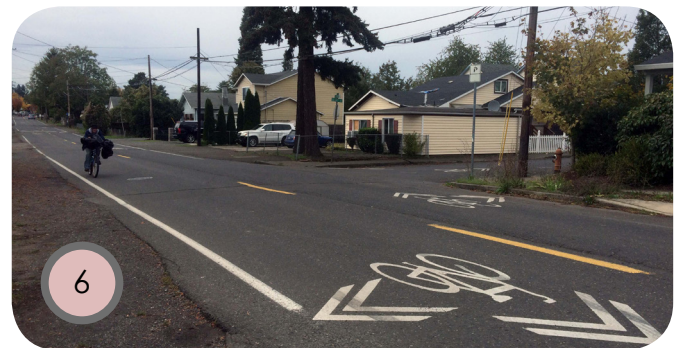
6 Difficult crossings on 87th and jogs in the route are weak links along this otherwise low-stress neighborhood greenway.
