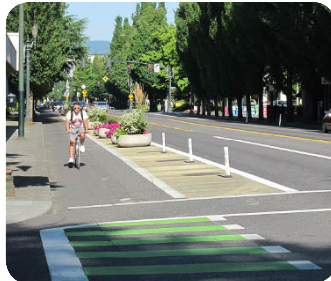
Planters can be used to protect cyclists. (Source: FHWA)
