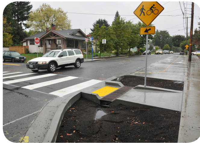
NE 33rd and Going St. looking north at a bulb out that reduces the crossing distance for pedestrians. (Source: BikePortland)
