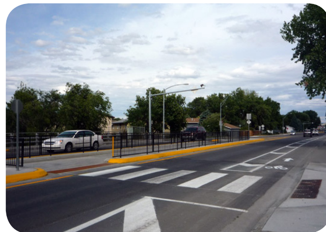
Center refuge island provides protected connection to an offset trail for a jog to the right, Billings MT (Source: NACTO)
