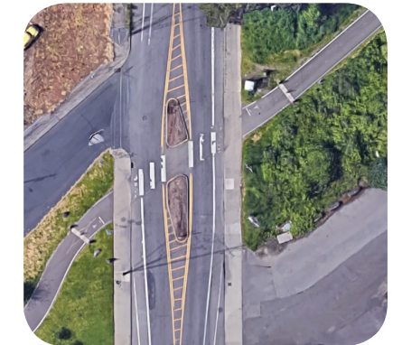
Bird's eye view existing conditions at 92nd & Springwater Corridor
