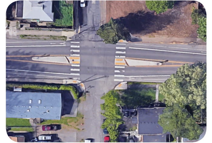
Bird's eye view of the current conditions of the intersection (Source: GoogleMaps)
