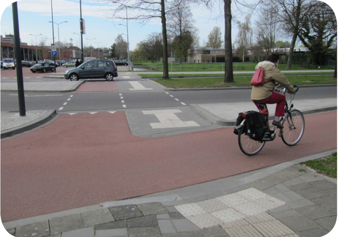
Crossing for the sidewalk and adjacent one-way protected bike lane in the Netherlands
