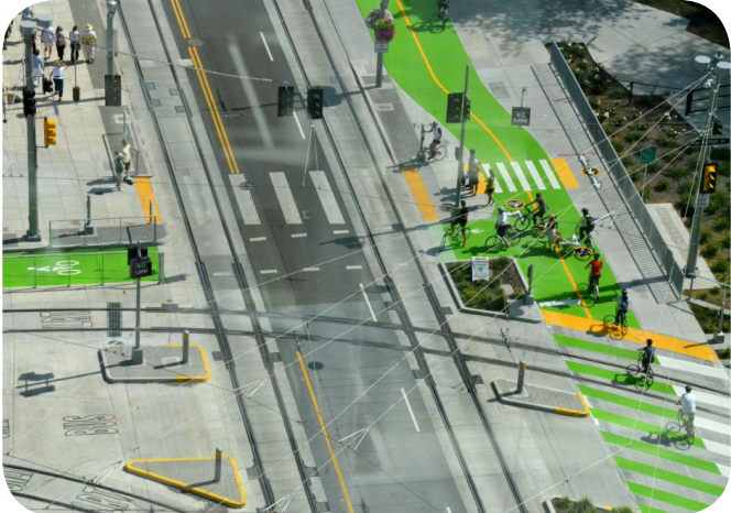
Left turn queue space and a bioswale on the Southwater Front in Portland OR
