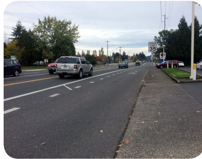
On Holgate Blvd (~15,000 ADT) to the east of 92nd the speed limit increases from 30 mph to 35 mph.
