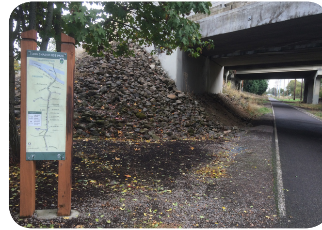
Existing underpass and signage on Springwater Corridor (Source: Author's analysis)
