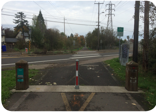
Existing crosswalk and pedestrian island at Springwater Corridor and Flavel (Source: Author's analysis)
