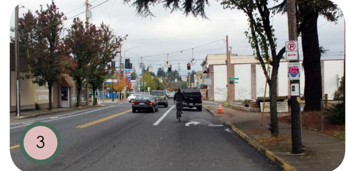
3 The narrow (~3.5-4 ft) bike lane on 92nd Ave. (~12,000 ADT) going northbound ends just prior to intersection with Woodstock Blvd. to create a right-hand turn lane for motor vehicles. No signs indicate that the bike lane will end or that bikes will be mixing with auto traffic.
