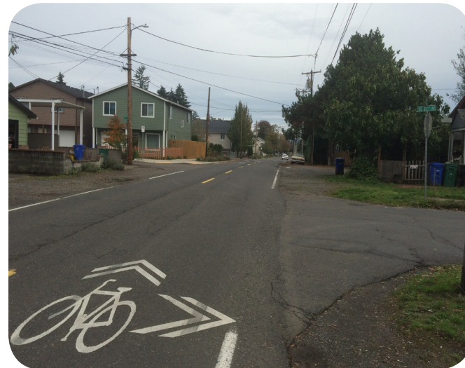
Missing sidewalks are more common further east.
