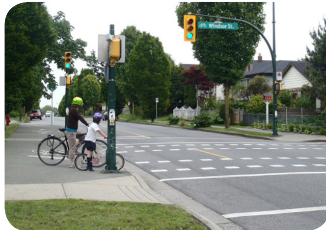
Two-way cycle track connecting a bike boulevard on Windsor St. for a jog to the right, Seattle WA (Source: NACTO)
