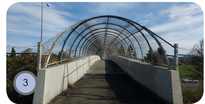
3 The Steele St bike-ped bridge provides a low-stress, east-west connection between residential areas, Lents Park, and Oliver Lent School.
