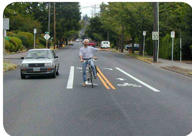
Center left turn lanes on SE Stark and 41st for a jog to the right, Portland OR (Source: NACTO)
