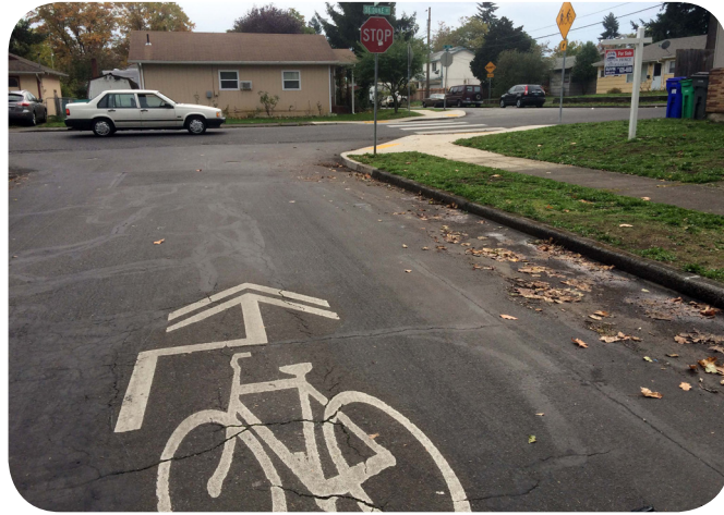
Looking south on 87th Ave
